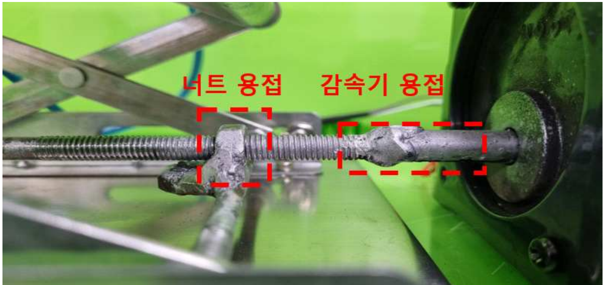
Fig. 16 Lead screw construction welded at the bottom of the lift
